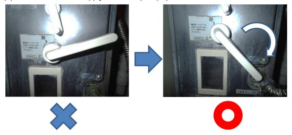
(7) Turn the hot water supply lever to "OFF (止)".
